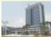
도청 provincial government building
